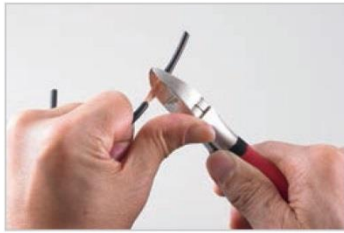
① 피복탈피 (Wire Stripping Operation)
